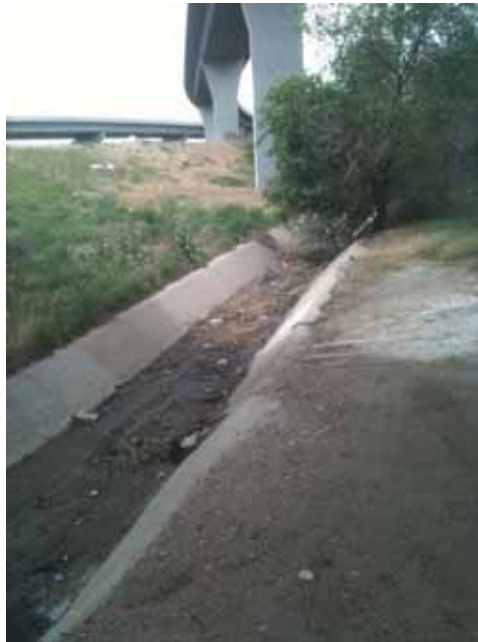
Photo 11 — The concrete lined ditch north and east of US 6 and I-25. No wetland plants or hydric soils are present; it is just filled with trash and mud.
