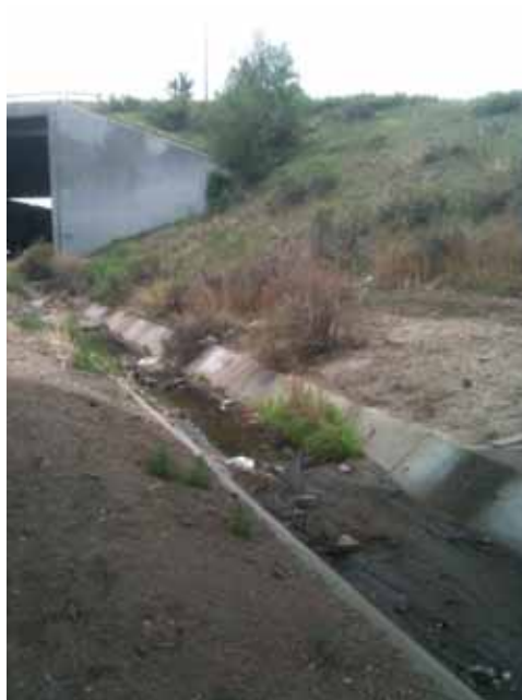
Photo 12 — The concrete lined ditch north and east of US 6 and I-25.
